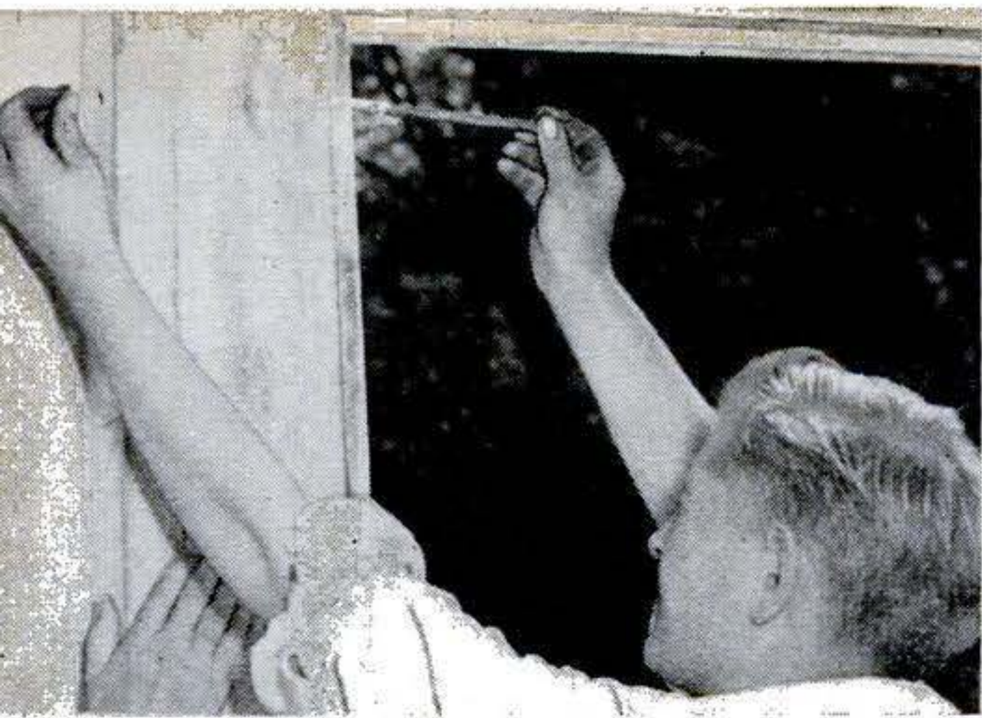
BOLTS THROUGH EDGES tie each wall section to the next one (left above). Bottoms are anchored by lag screws into wooden sleepers
